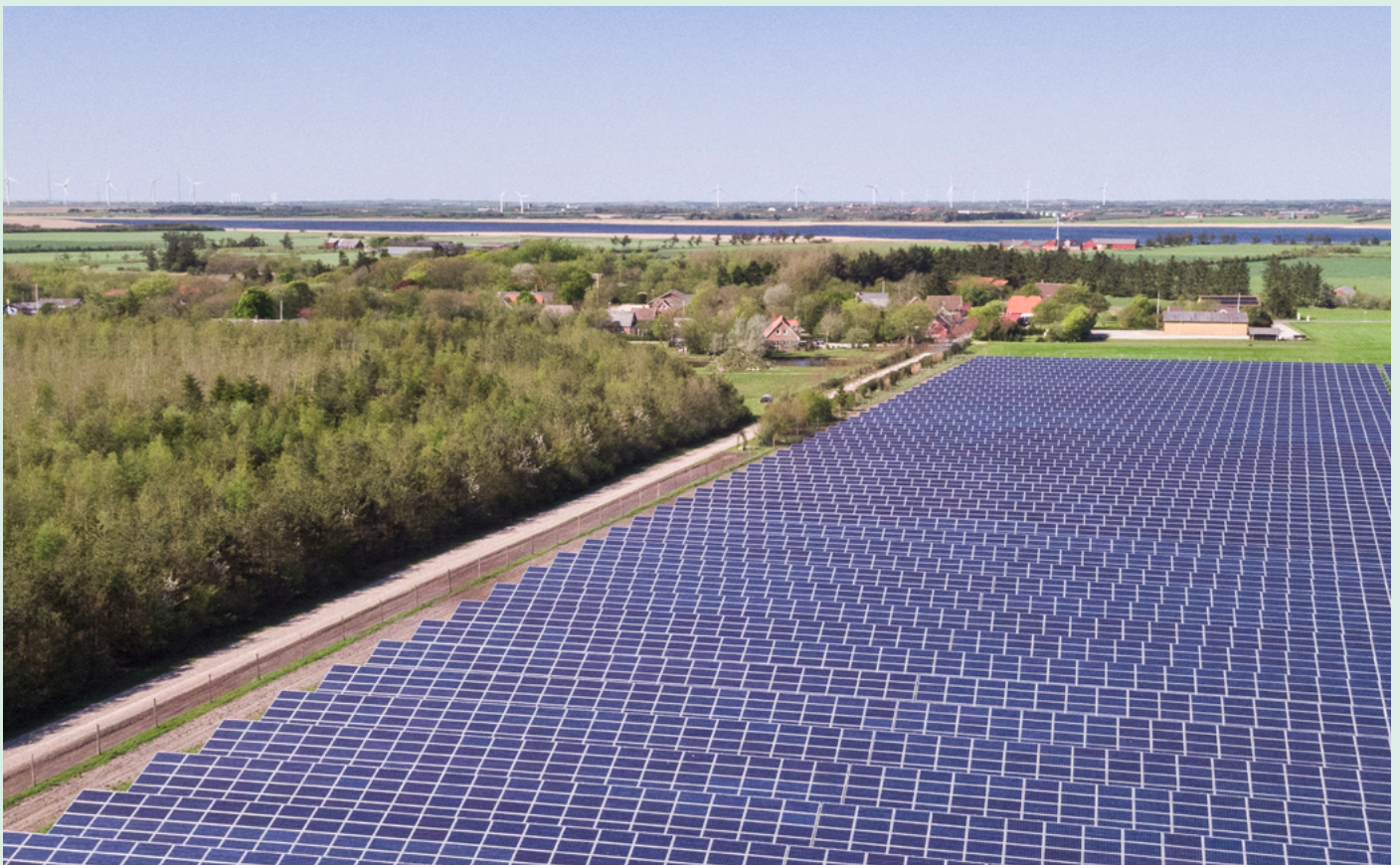
NRGi Solcellepark Nees
